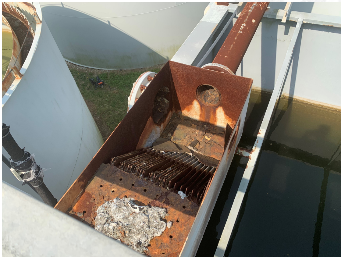
Package WWTP Bar Screen
