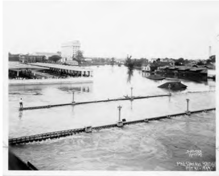
Preston Ave Bridge, 1929
